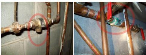
Observation: The "Air Vent" mounted on top of the "Purger Valve" at the boiler is corroded or drip leaking.
