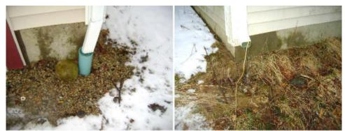
Observation: The downspouts empty roof run-off water near or adjacent to the foundation.
