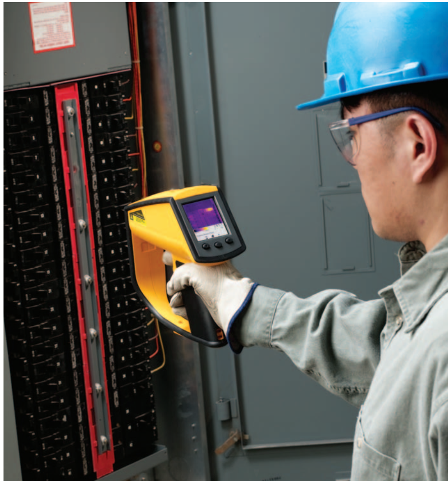
Use thermal imagers to check energized components for hot, loose or corroded connections.
