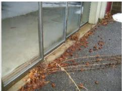
Observation: The door jambs at the exterior door are rotted out at the basement entrance.
