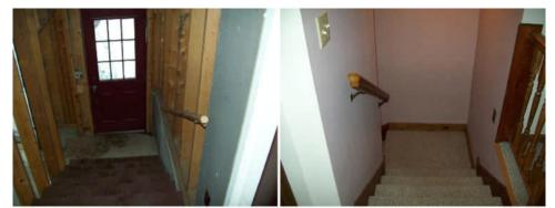
Observation: The staircase to the basement and second floor lacks returns at each end of the handrail.
