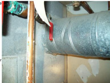
chimney wall designed to accept the flue connector from an appliance. They must be placed with the chimney end flush with the inside wall of the flue lining and cemented in place with the refractory mortar used in the flue tiles.
