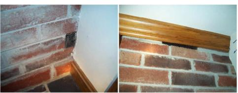
Observation: Unplugged openings are present in chimney. In the basement the insulation is not an appropriate means to plug a flue. Also in the first floor there are what appear to be vents in the brick work.
