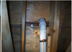
Observation: The flashing and/or the rubber gasket around the plumbing vent pipe appears to be defective.
