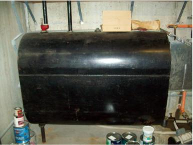
advise than any oil tank 30 year of age or older be replaced as a precaution against leakage, environmental contamination and uninsured major expenses for cleanup. For your budget, to have an old tank removed and a new one installed costs between \$1200 and \$1500. Replacement should also include any old oil line that is not enclosed in a protective sleeve that shunts any oil leakage to the head of the pipe where the homeowner can see the leakage.
