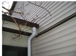
Observation: The joint between the stoop and the house siding does not appear to be flashed
